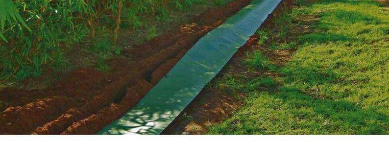
Plantex\* RootBarrier is the ideal solution to control plants with aggressive root systems such as bamboos and pyracantha. It is particularly recommended for critical applications such as protecting buried linear networks: cables, water piping, pavements, paved areas, roads, water and sewage networks.
